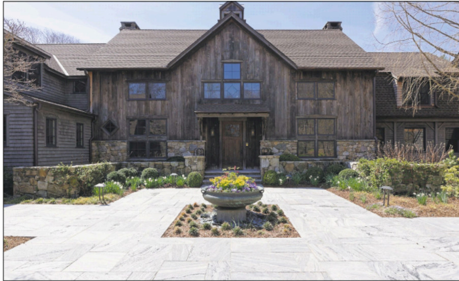
The converted chestnut wood barn at 279 North Ave. was originally built in Weston in 1832. It was modernized and expanded on its current site on the Aspetuck River by renowned local architect Michael Greenberg in 2000. Contributed photos
