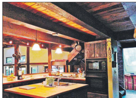
As seen here in the kitchen, the structure is held together by its original chestnut beams.
