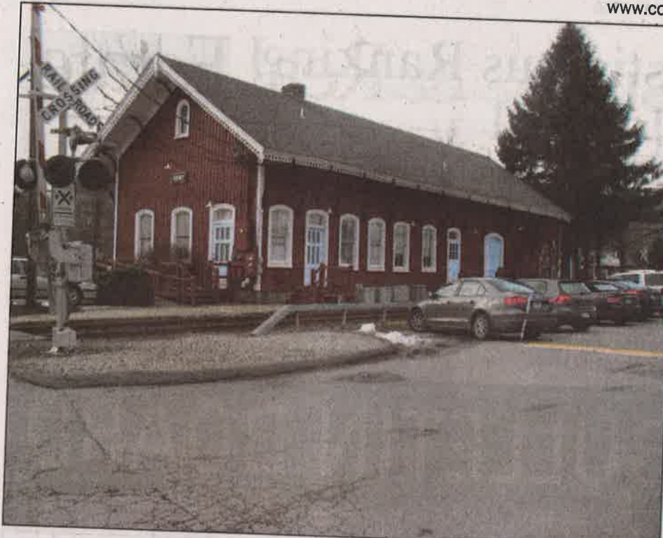
The Kent Railroad Station.
