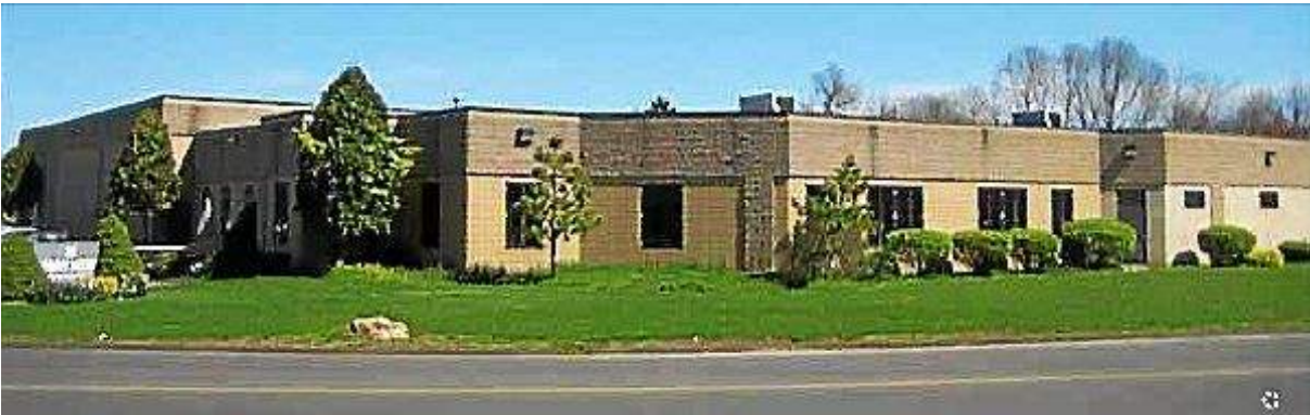
16 Business Park Drive, Branford
