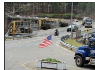
Stevenson Dam repairs require road closure
